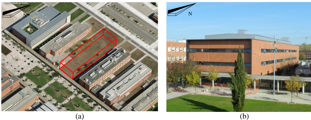
Figure 6.2 – Case study: (a) location in the Aveiro University Campus (b) built department building
