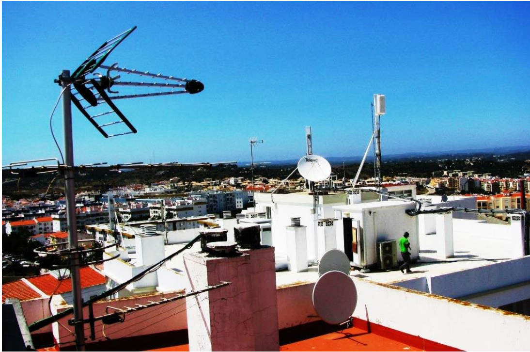
Fig. 4.25. The interferer tri-axial Yagi-Uda aerial.
