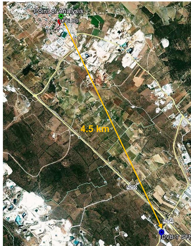
Fig. 4.18. Relative positions of the receiver, the LTE BS and the DTT best-server transmitter.
